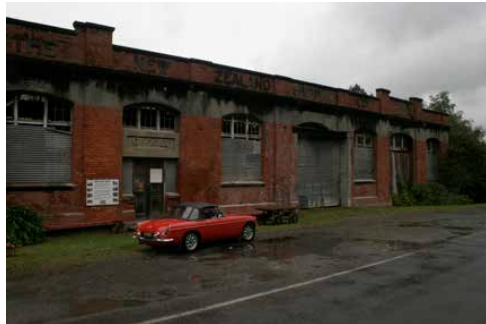
Derelict building Tokomaru Bay
