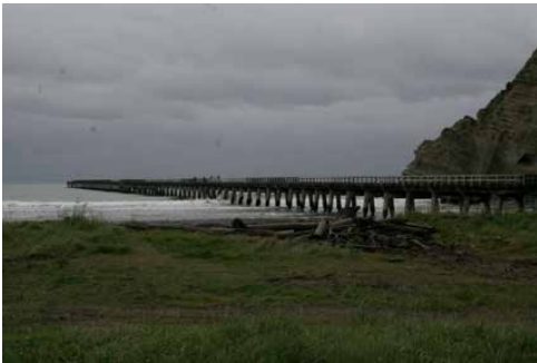
Wharf at Tolaga Bay
